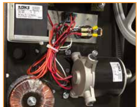
dc motor and battery backup for continued gate operation if AC power is lost
